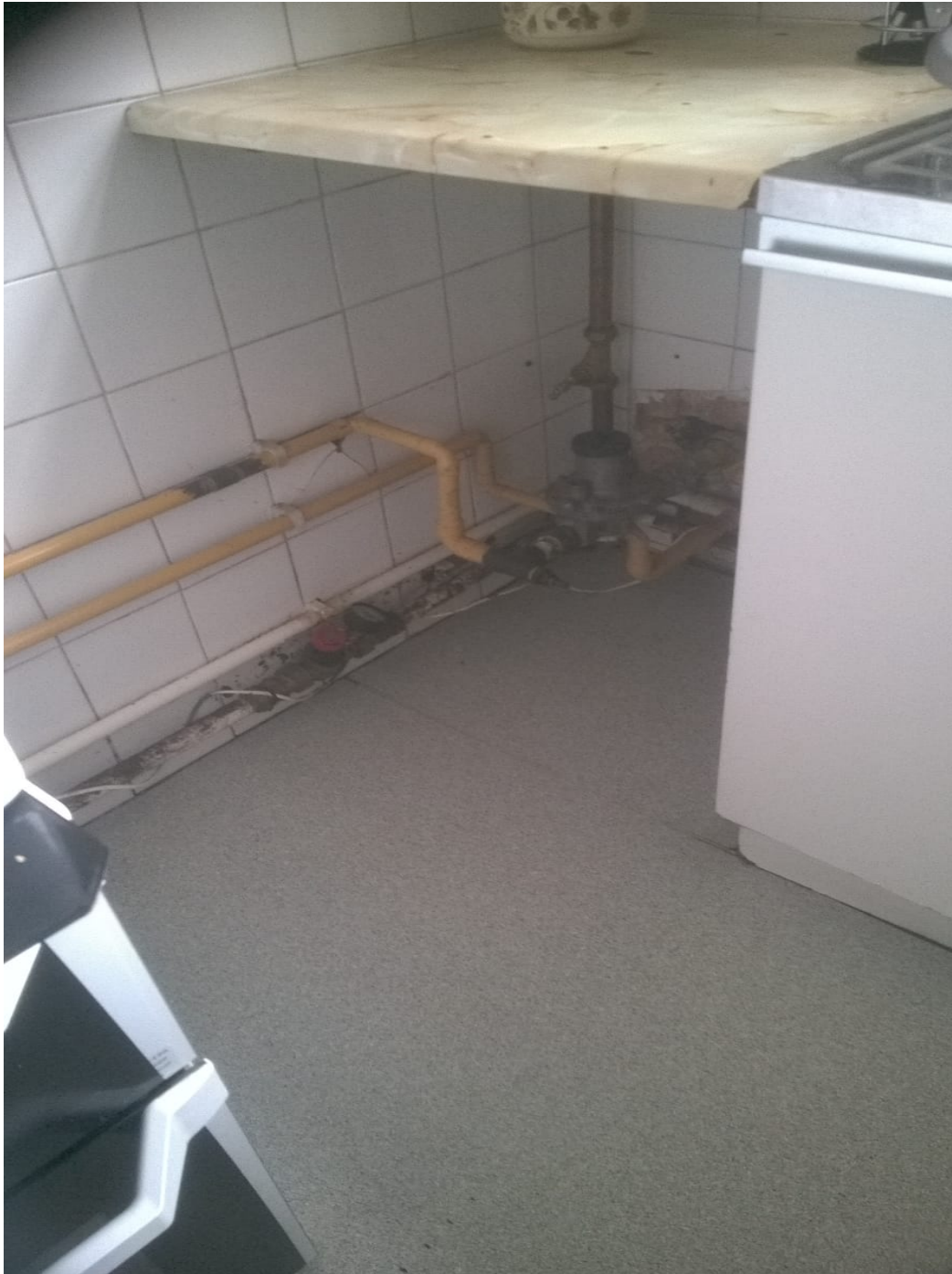
Kitchen (main building) This to be sectioned off after the works completed
